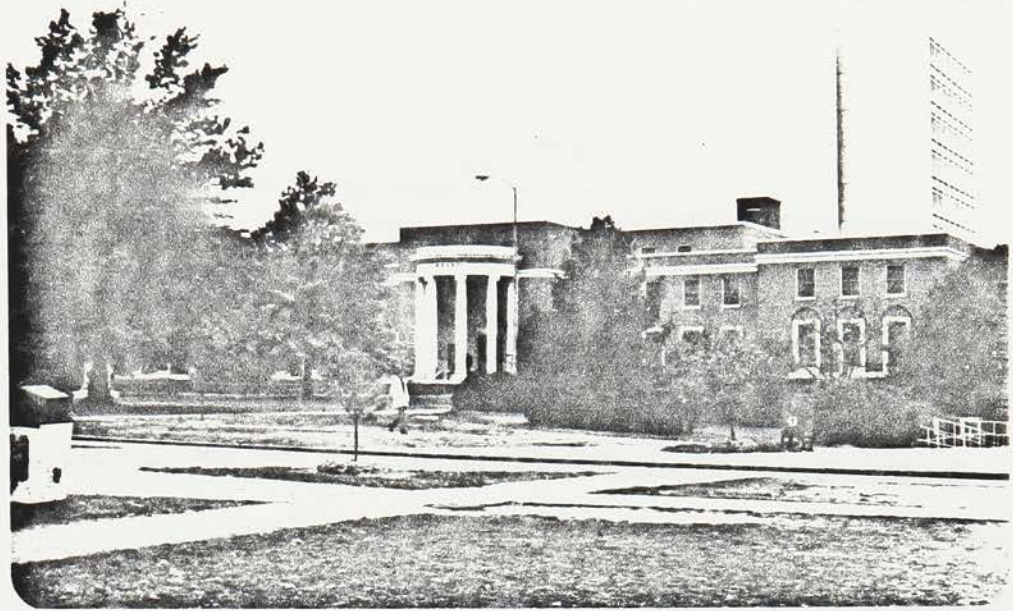
The Walter Clinton Jackson Library is one example of the changing vista on campus. The original wing was built in 1953 with the ten story addition added in 1973. The library contains over one million volumes and has a variety of seating locales.
