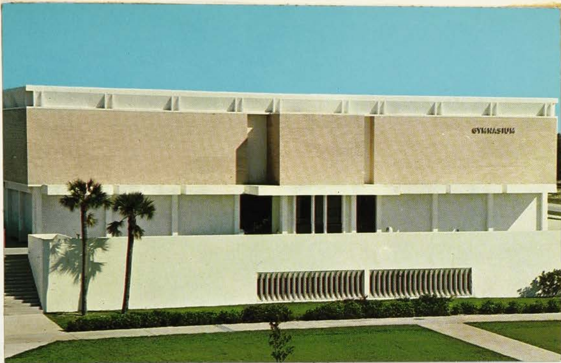
PHYSICAL EDUCATION CLASSROOM BUILDING, housing the director and faculty of the Division of Physical Education, classrooms, gymnasium, activities area, and an indoor swimming pool
