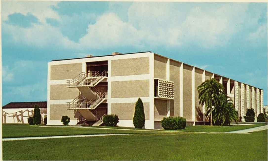
Chemistry Building, University of South Florida, Tampa, Florida
