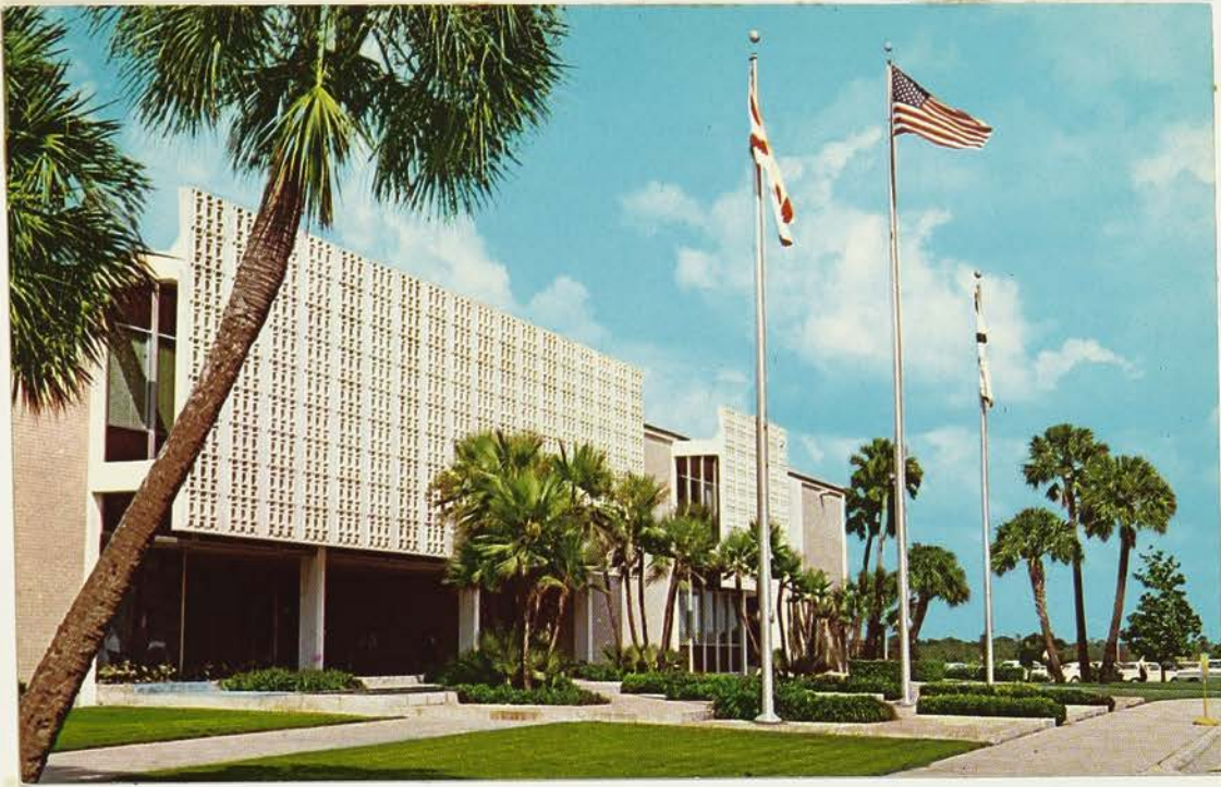
ADMINISTRATION BUILDING, housing administrative and business offices and a number of special service units of the institution.
