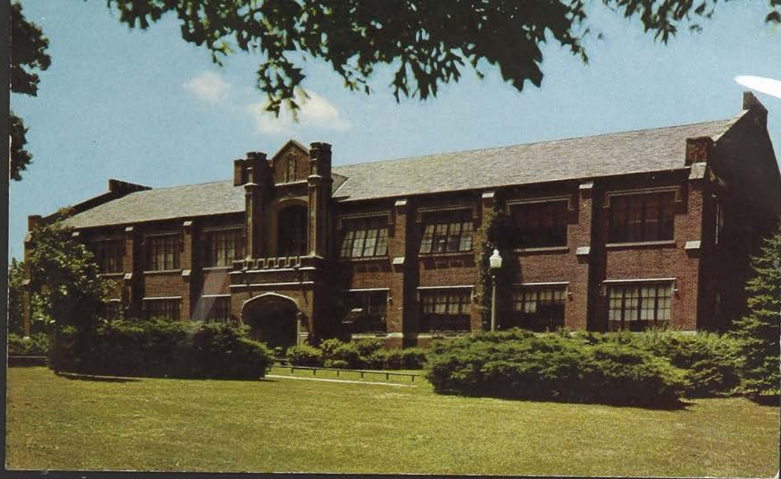
ENGINEERS BUILDING AT ROSE POLYTECHNIC INSTITUTE
