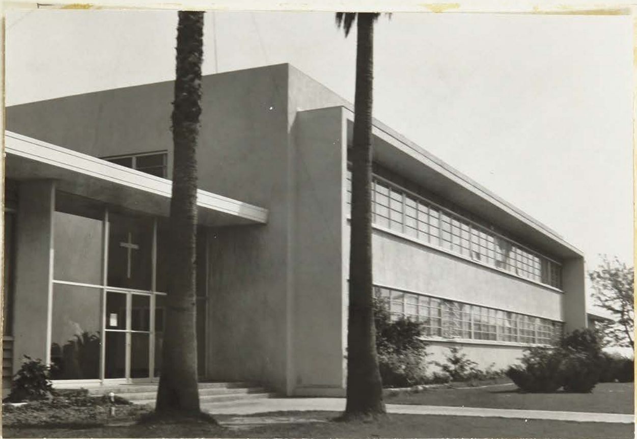
Pereira Hall, Engineering Building
